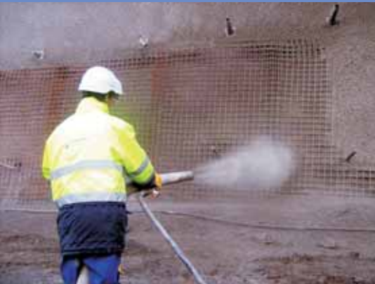
LGV - Tunnel de Chavanne - 25
